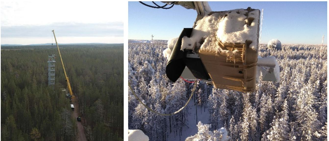
*Figure 8. Installation of microwave equipment in ICOS tower at FMI-ARC in Sodankylä, Finland, in the summer of 2018 (left). SodScat radar overlooking the boreal forest test area in the winter of 2018-2019 (right).*
